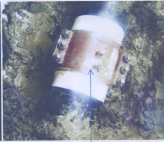
Picture of the 2mm hacksaw cut on the facility (before and after clamping)
